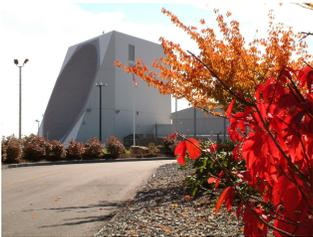
The Pave PAWS main building is shaped somewhat like a pyramid with a triangular base 105 feet on each side. The two array faces, each containing 1,792 active antenna elements, are tilted back 20 degrees
